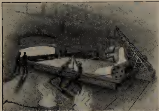
FIG. 153. Casting and rolling plate glass
